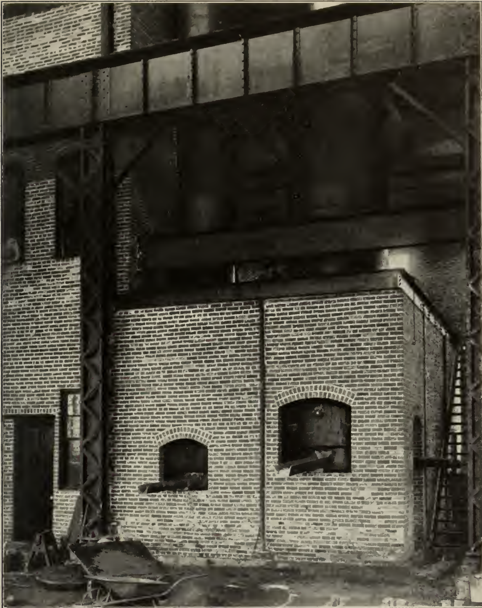
NEWTEN CUPOLAS, FOUNDRY OF DETROIT SHIP-BUILDING COMPANY.
